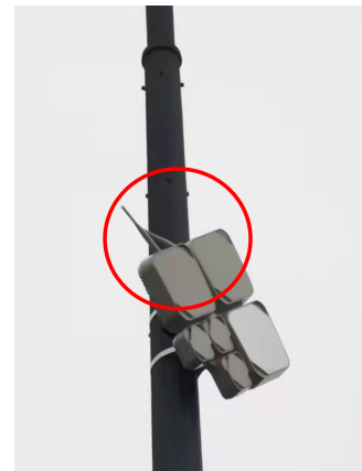
FIGURE 20: Loose external antenna and misalignment after a few months of deployment, causing connectivity problems.
